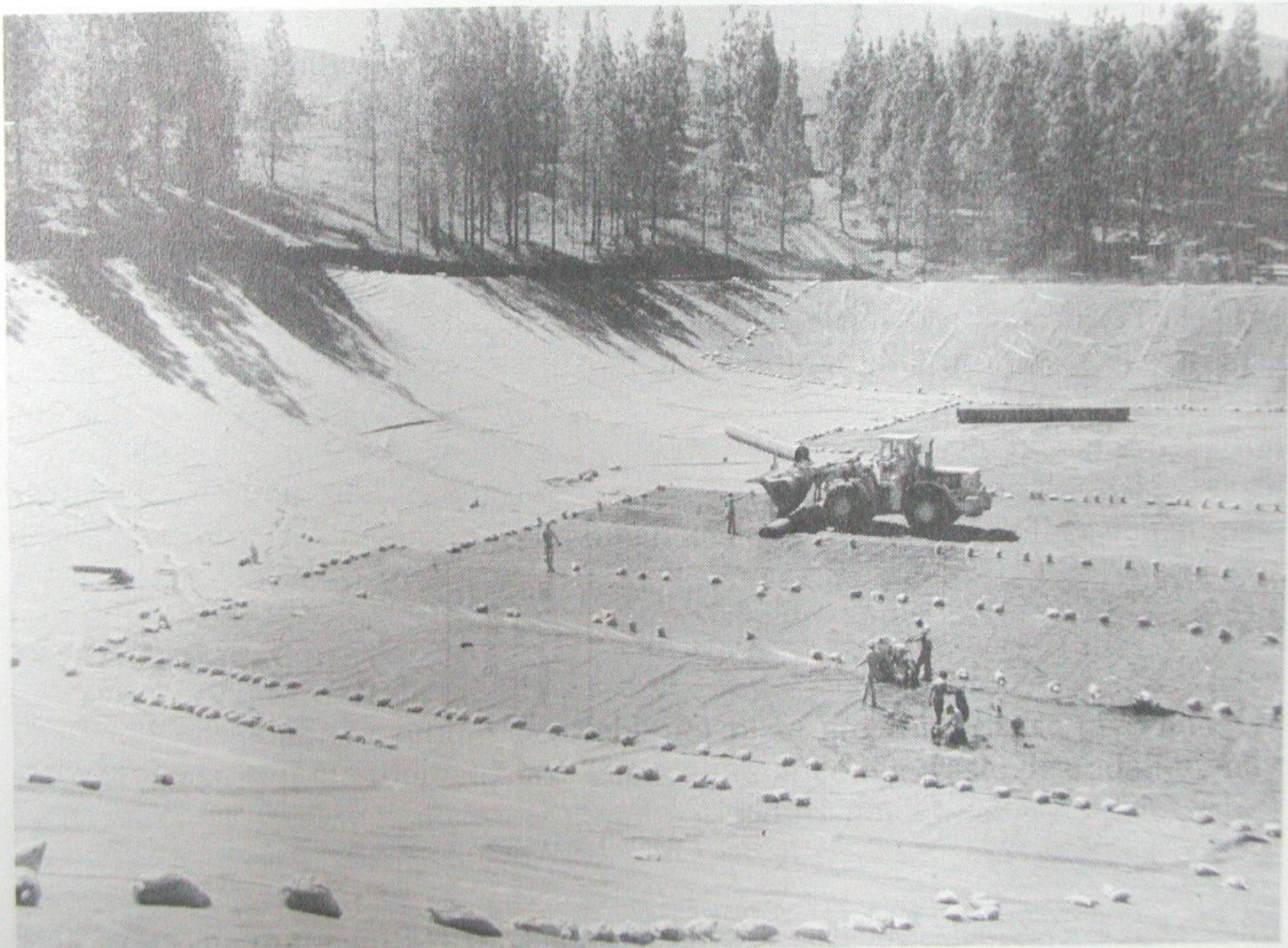
FIG. 10.2.3 Installation of an FML sheet
