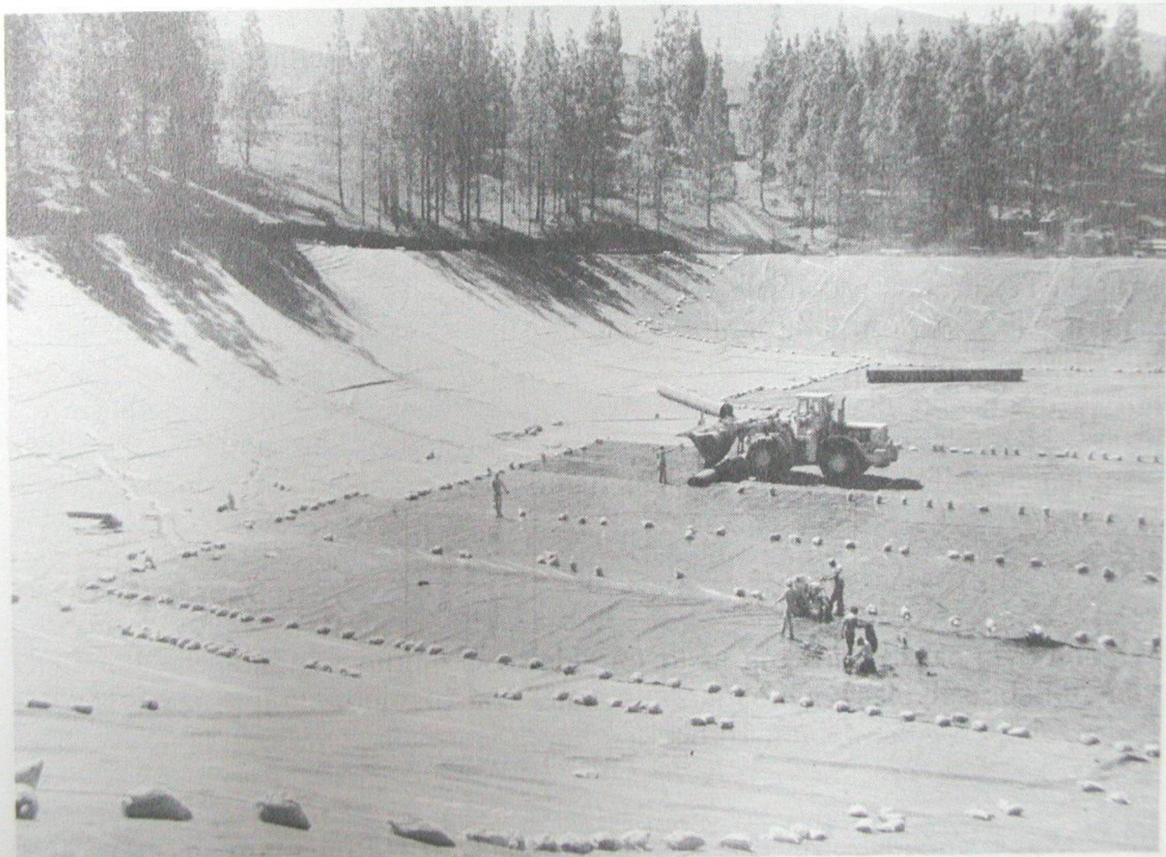
FIG. 10.2.3 Installation of an FML sheet
